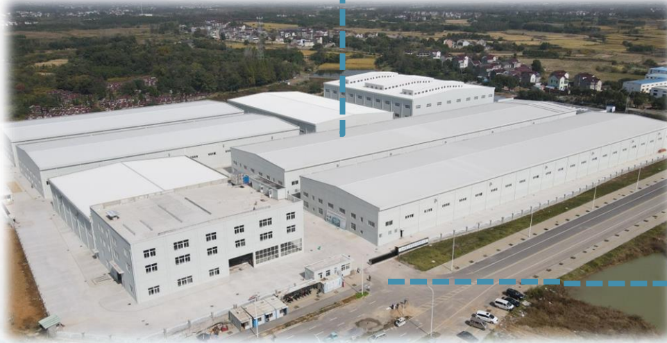
Photo of new Anhui plant site
