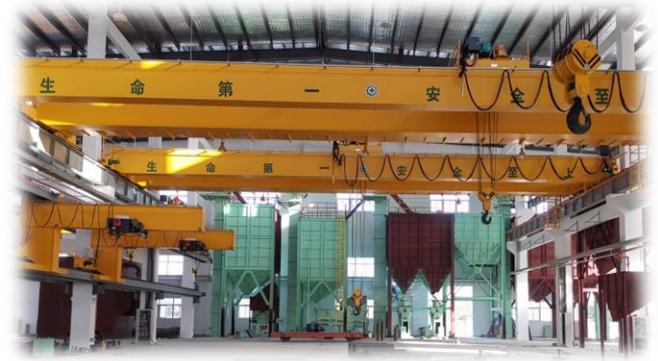
Molding Workshops Equipment Installation
